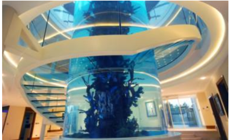
This three-story aquarium collapsed when two vertical seams opened unexpectedly. Image: The Sun, U.K.
