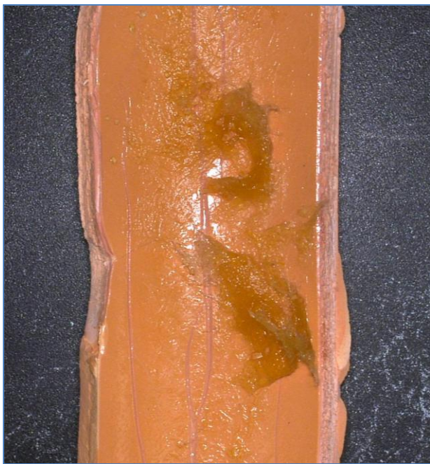
Figure 11 – Material observed at inner surface of failed CPVC pipe exposed to a mixture of water and bio-glycerin.
